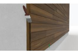
When the head parts of the cladding are cut off, it is absolutely necessary to apply preservative to the cut head parts.
